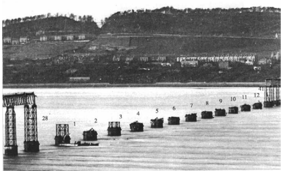
Figure 29.4 Fallen piers as seen from the south bank of the firth. For the purposes of the investigation, the piers between 28 and 41 were renumbered 1 to 12.
